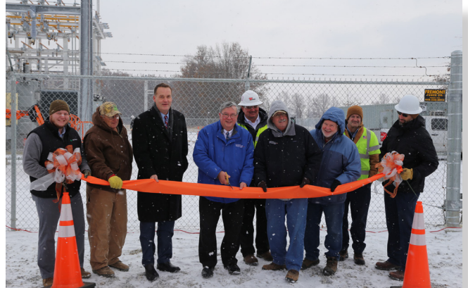
Ribbon Cutting: North Central Electric completed construction on the Adrian substation in northeast Wyandot County. It is the cooperative's 12th substation, and first since 2002.
